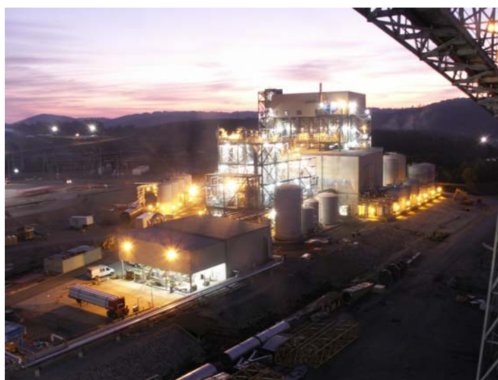
Figure 7-3: DuPont Tate & Lyle Commercial Bio PDO facility at Loudon, Tennessee
