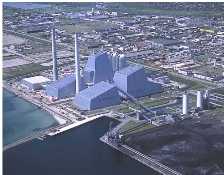
Figure 4-5: Avedore 2 Combined Heat and Power Plant
