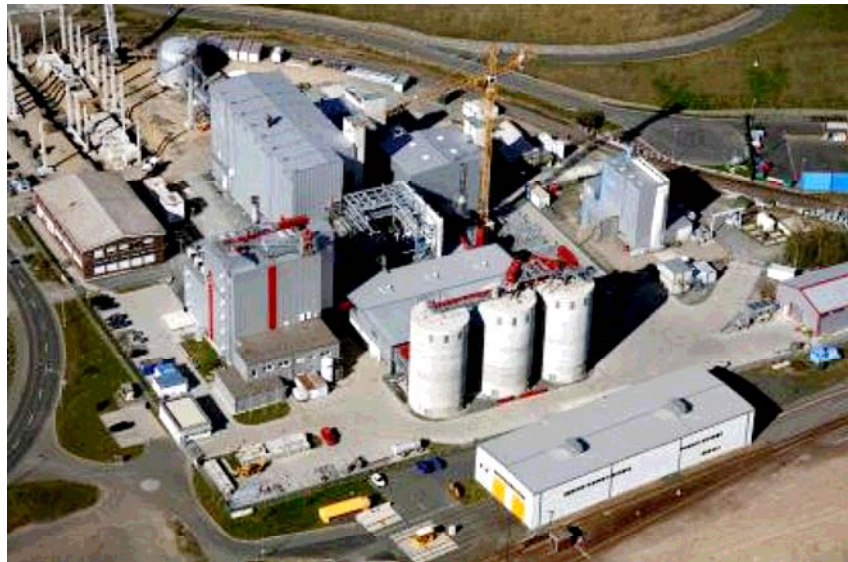
Figure 6-4: Choren BtL plant under construction at Freiburg, Germany (source: Choren)
